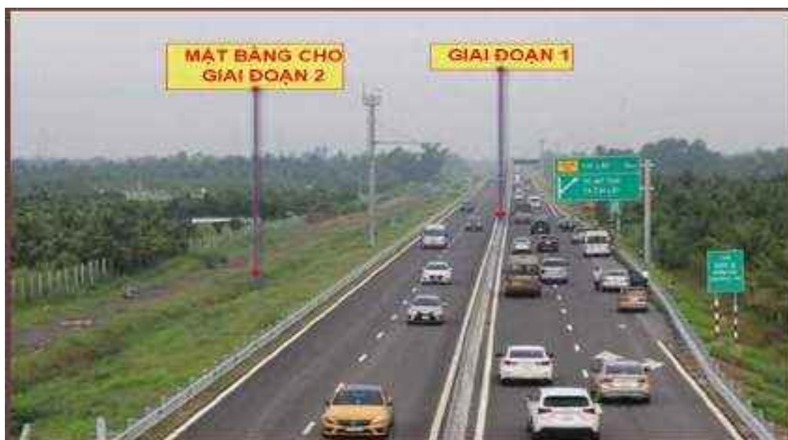
Figure 2: Current status of the Trung Luong – My Thuan section
